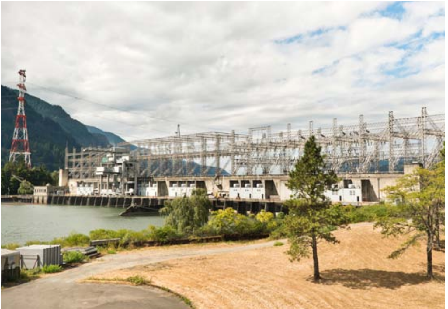
POWER GENERATION AT BONNEVILLE DAM IN OREGON
